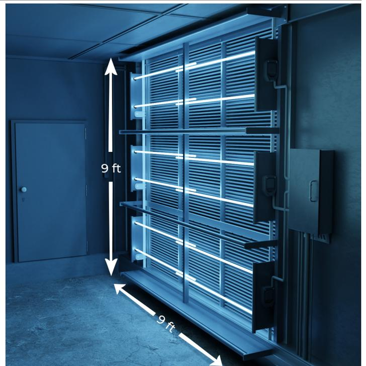
Until recently, low-pressure mercury vapor or fluorescent UV-C lamps have been the best option for disinfecting the cooling coils in AHUs. These lamps are low intensity, must run continuously (24/7) and be mounted at a close distance (4"-6") to coils and filters.
